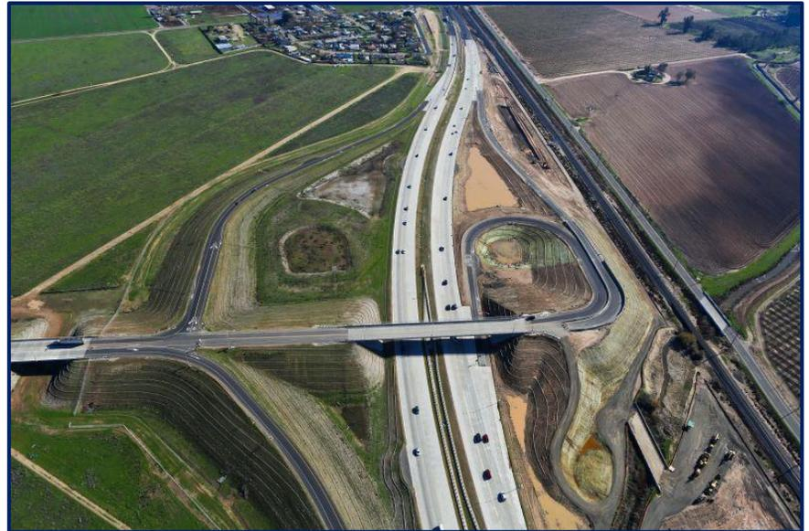
**Completed:** Phase 1A was completed in 2016. It replaced the Buhach Road ramps with a modern interchange, upgraded a mile of SR-99, and constructed Green Sands Avenue and the first portion of the AME as a two-lane facility. It cost \$66 million, including \$19 million from MCAG impact fees and regional transportation funds, and \$47 million for construction from the state’s 2006 bond.
